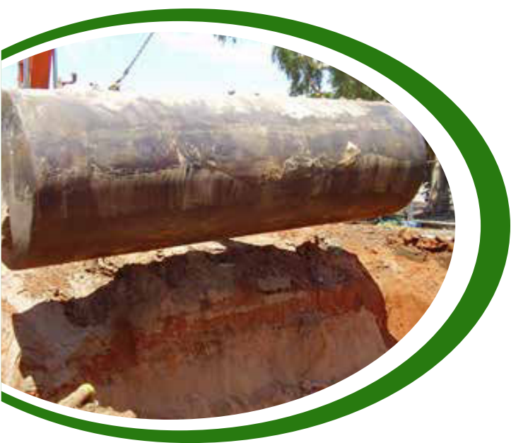
Figures 7 & 8. An underground fuel tank being removed.
